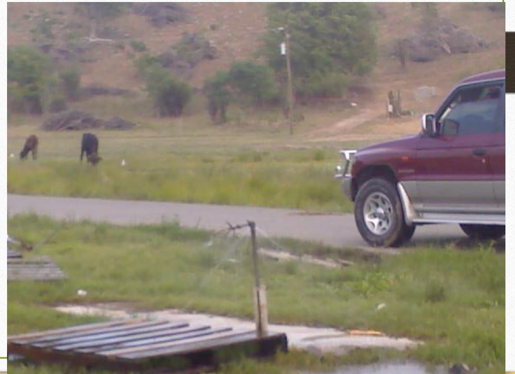
Stand Pipe at Ffryes
