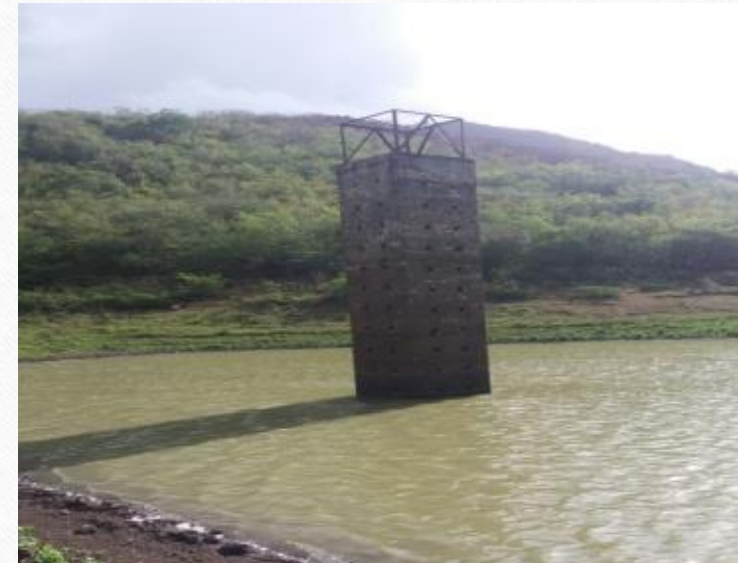
Pot Works Dam, May 2016,
