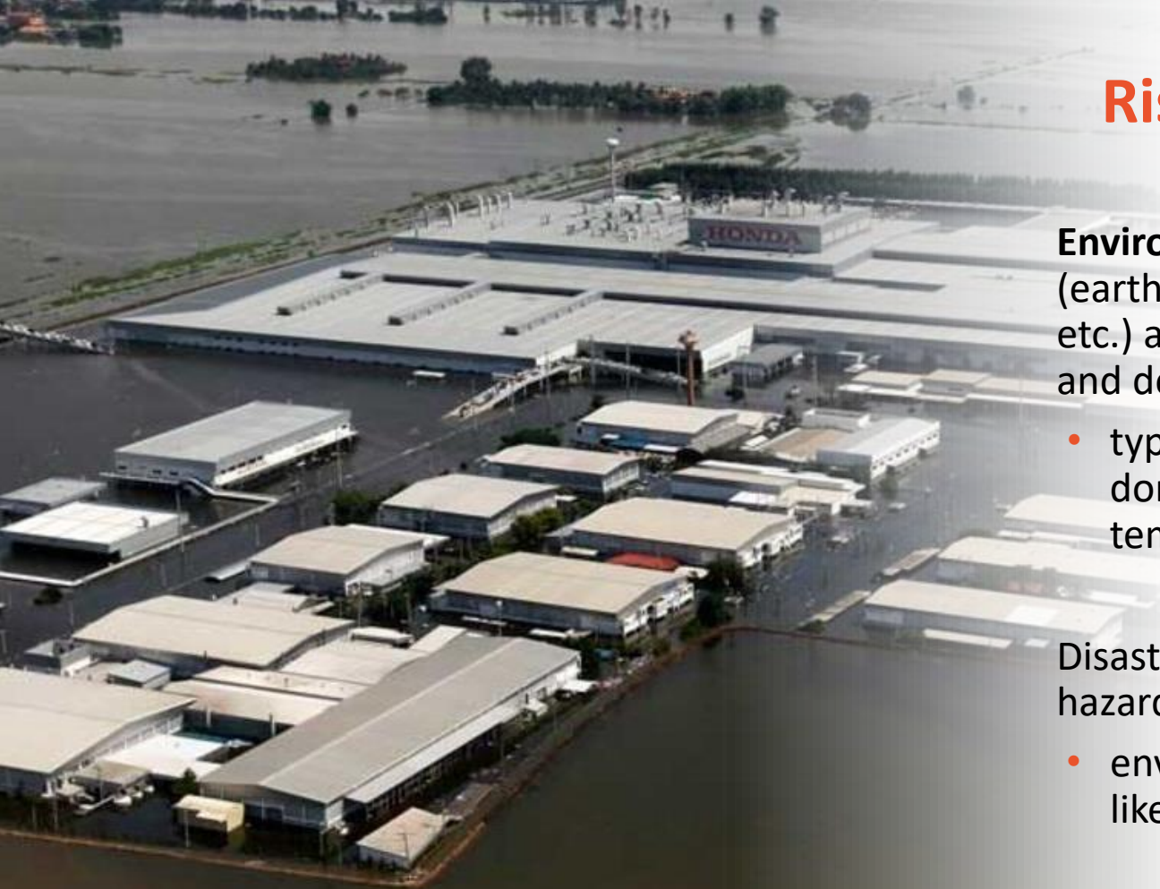
Honda car factory in Ayutthaya province, Thailand, during the 2011 floods.
